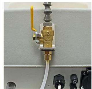
7. Attach tube into Glastar Machine and tighten nut with a small spanner (not supplied).
